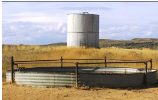
12,000-gallon storage tank and watering tank in Section 32.
