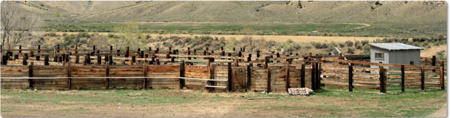
Wooden livestock corrals & windbreaks were re-constructed in 2006 and include a 20,000 lb. livestock scale.
